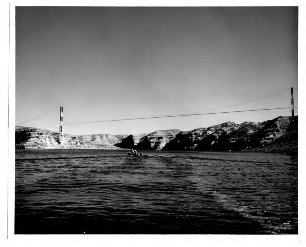
In this photo may be seen part of the suspension bridge built to carry a twenty-six inch high pressure natural gas line across the lake. This gas line carries natural gas from the Four Corners in the southwest to the Pacific Northwest.
