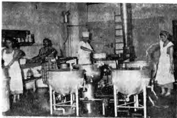
Section of main kitchen. Fast working steam kettles cut labor requirements to minimum. Electric dumb waiters deliver bulk food to floor pantries. A special diet kitchen is on an upper floor.
