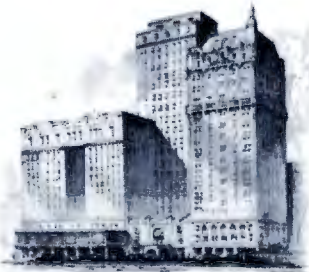
OWNED AND OPERATED BY THE DALLAS HOTEL COMPANY
