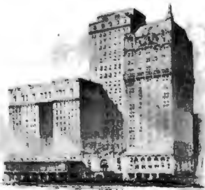
OWNED AND OPERATED BY THE DALLAS HOTEL COMPANY
