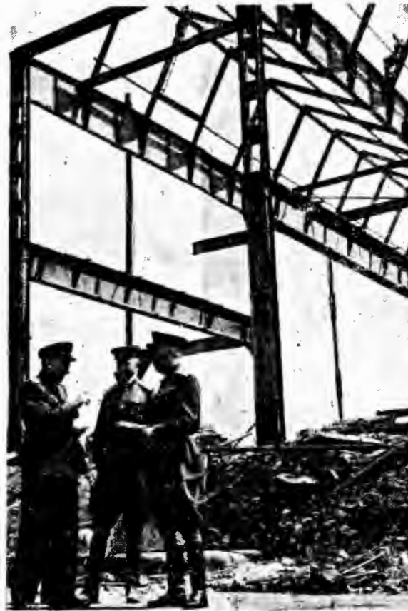
Russian officers talking at Siebel Plant where steel girders are being removed.
