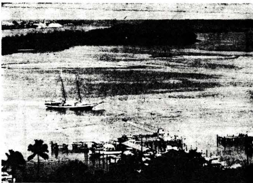
UGLY new mud island in Biscayne Bay can be seen across the center of this picture. They were thrown up by pipeline dredges digging the trench for a cross-bay sewer main.
