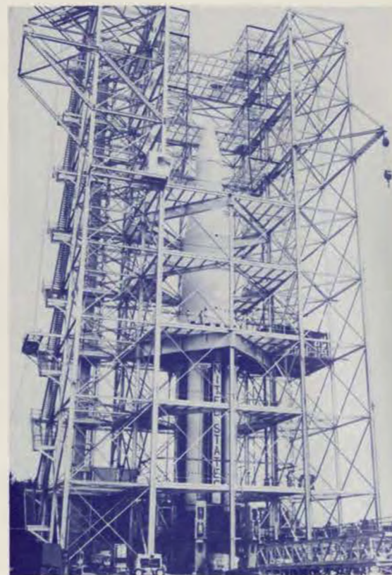
Full-scale model mockup of Block I vehicle undergoes vibration analysis in this dynamic test tower at MSFC to insure perfect engineering in the flight models.
