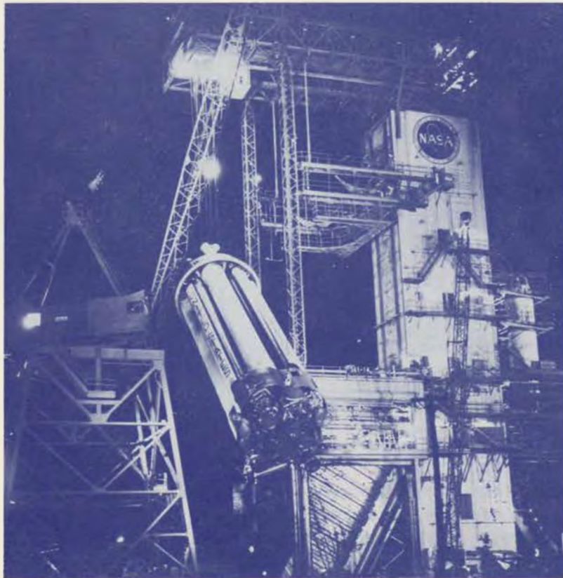
The first Saturn S-I stage being installed in the static test tower at MSFC. Here the rocket underwent captive firing tests to insure reliable performance.
