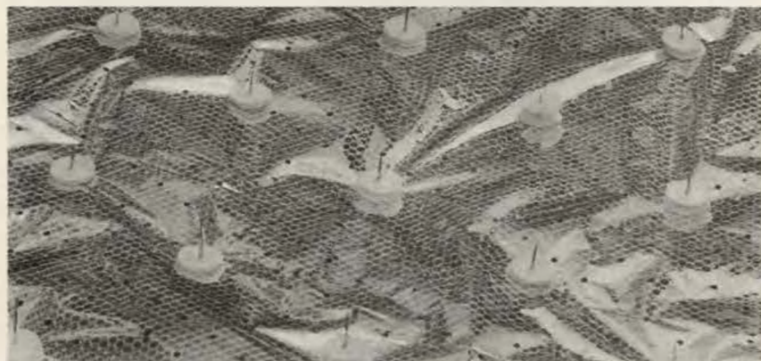
Multi-layer insulation pinned on the wall of a tank.
